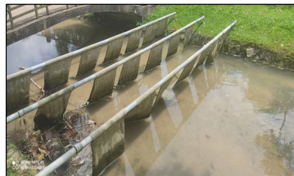
(b) NWG were arranged in 3 rows across the river at TPBKKL intake pond.
