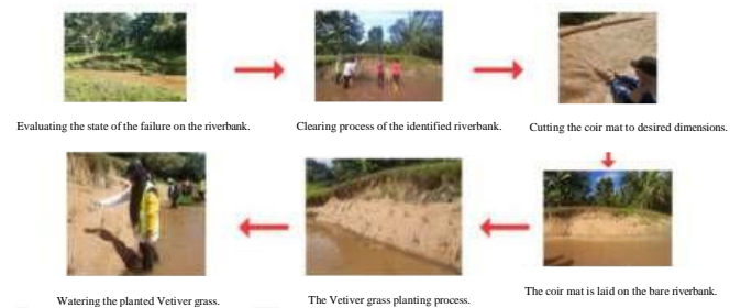
Fig. 4 – Step by step of the installation of sustainable riverbank protection
